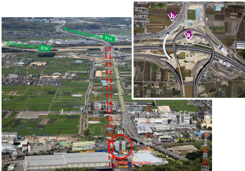
JOYO Viaduct, Shin-meishin Expressway Project by NEXCO West
